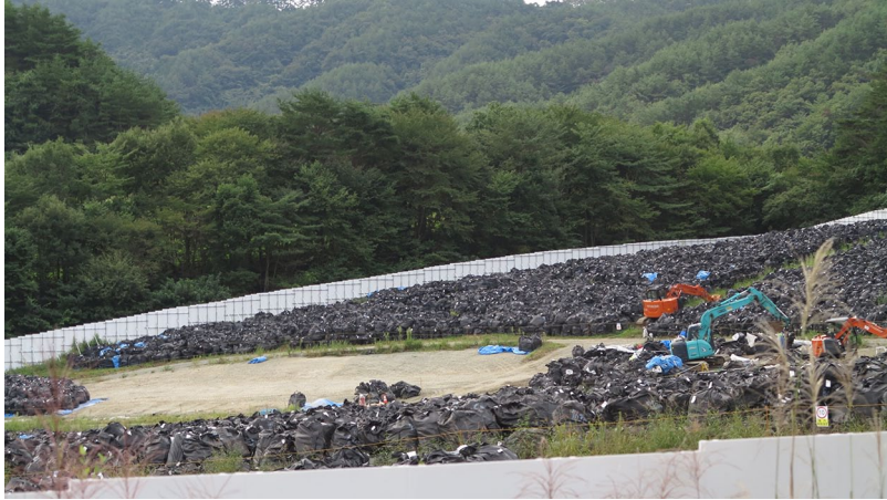
Figure 2. A temporary site of radioactive waste disposal in Iitate, Fukushima. After the nuclear disaster, radioactive tainted soil and debris have been put in vinyl bags. These bags are kept in temporary storage spaces and there is still no long-term solutions concerning their disposal (photo by the author).
